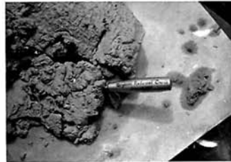
Work on the stone
