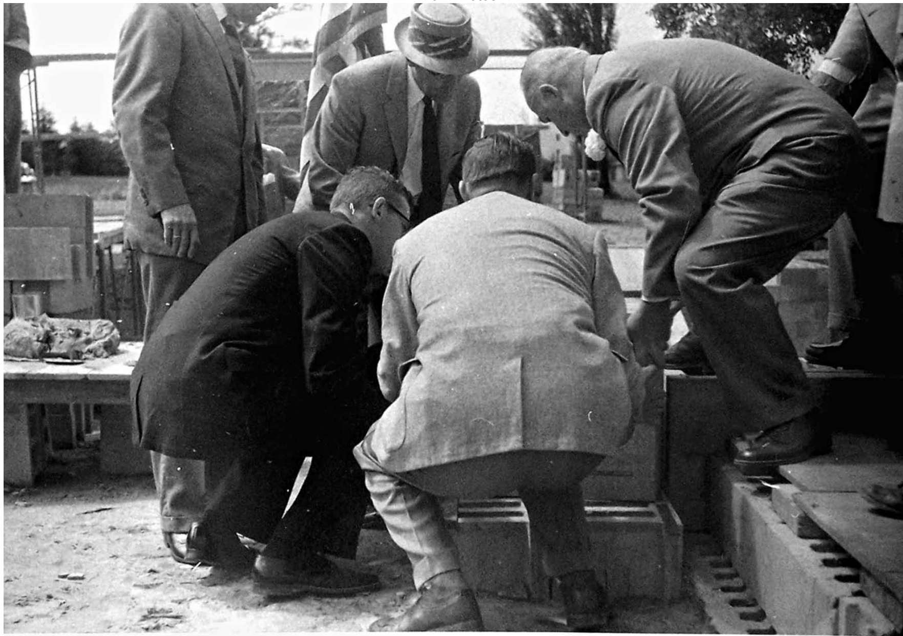
Putting corner stone in place 4 men not identified
