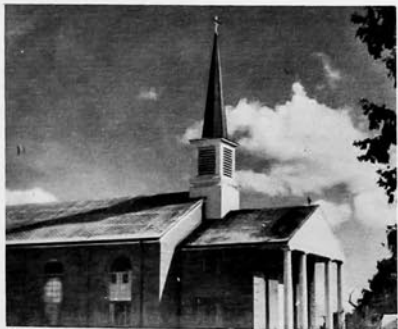
A contemporary colonial building. The steeple was all built and then raised into place with a derrick.
